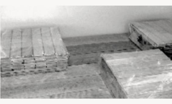
4. When gluing, it is important that the planks are continuously weighted during installation to ensure optimal adhesion to the subfloor. HØRNING MS Flexlim III Eco must dry for 48 hours before sanding and surface treatment can begin.
