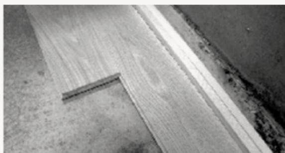
4. Alternatively, a stop strip can be screwed to the subfloor (one plank width + 10–15 mm from the wall); the first row is then laid last, ensuring a straight line against the wall.
