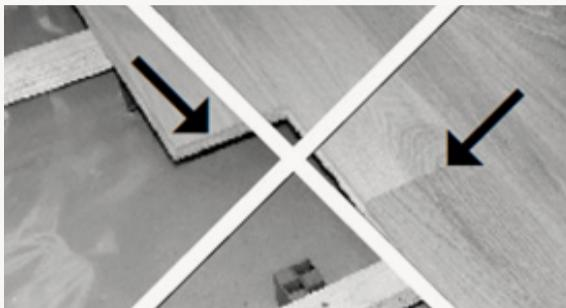
4. Avoid flying joints as much as possible; joints must not be in the same joist bay and must be at least 600 mm apart. There must be at least two continuous planks after each flying joint.
