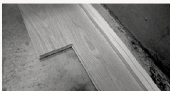
2. Alternatively, a stop strip can be screwed to the subfloor (one plank width + 10–15 mm from the wall); the first row is then laid last, ensuring a straight line against the wall.
