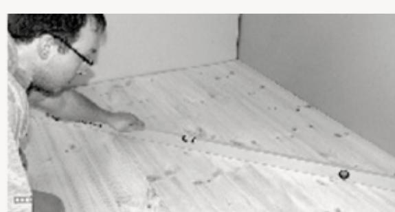
2. The subfloor must be level  $\pm$  2 mm per 2 m, measured with a straightedge. For uneven floors: plane, level, or lay a board (chipboard or plywood).
