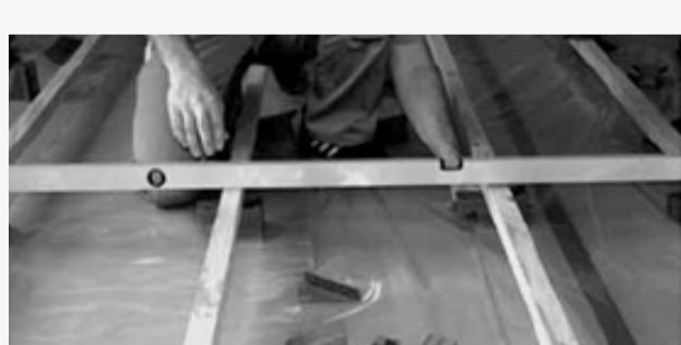
4. The joists must be completely level +/- 2 mm per 2 m.
