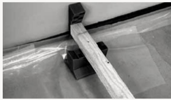
6. The distance from joist ends to walls should be approx. 10 mm.
