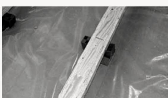
7. Joists that are joined must be supported by a chock and joined with min. 300 mm fishplates on both sides of the joist, e.g., fishplates of plywood 12 x 400 mm screwed with min. 12 screws in each plate. Furthermore, joints in the joist structure must be staggered to achieve a stable base. Remember to glue the joints.
