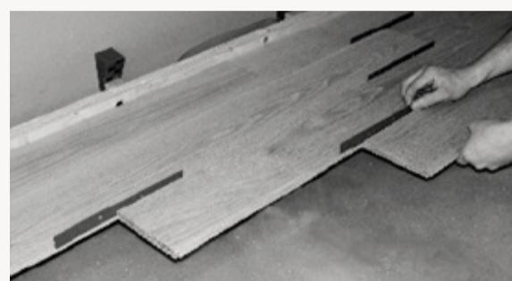
1. The 10-Plank Measurement must be observed, and spacers of 0.3 or 0.6 mm thickness can be used if necessary. This ensures the floor has room to expand during the humid season.
