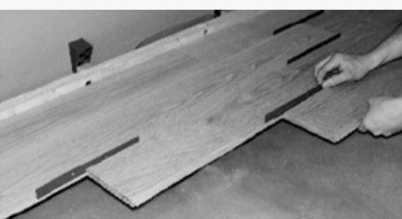
1. The 10-Plank Measurement must be observed, and spacers can be used if necessary. This ensures the floor has room to expand during the humid season.
