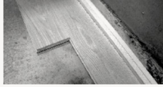
3. Alternatively, a stop strip can be screwed to the subfloor (one plank width + 10–15 mm from the wall); the first row is then laid last, ensuring a straight line against the wall.
