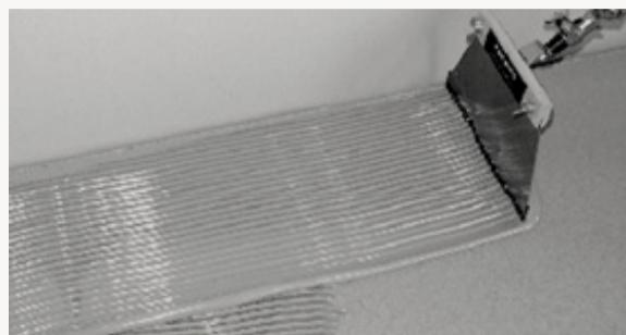
4. Apply HØRNING MS Flexlim III Eco using trowel no. 6. Approximately 1 litre per m<sup>2</sup> should be applied. Do not apply more adhesive than can be installed within 20 minutes. Installation must be carried out in wet adhesive. Adhesive must not be forced up between the planks, and tongue and groove must not be glued.
