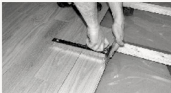
6. Always use a tapping block or crowbar. Be careful with the wall during installation.
