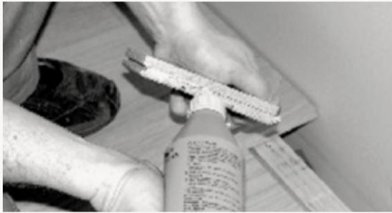
5. Always glue the end joints. Never glue tongue and groove. Do not glue on joists.
