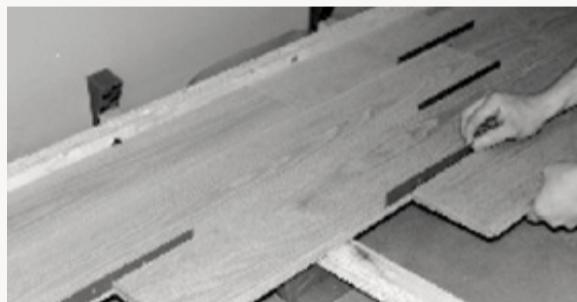
2. The 10-Plank Measurement must be observed, and spacers of 0.3 or 0.6 mm thickness can be used to allow the floor to expand during the humid season. You can choose to pre-drill and fasten the floor with floor screws instead of nails.
