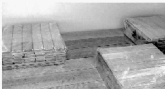
5. During gluing, it is important that the planks are continuously weighted during installation to ensure optimal adhesion to the subfloor. HØRNING MS Flexlim must dry for 48 hours before sanding and surface treatment can begin.
