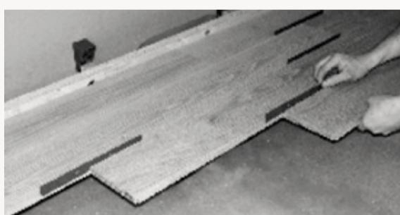
3. The 10-Plank Measurement must be observed to allow the floor to shrink and expand without displacement.
