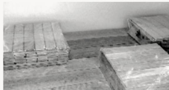
5. During gluing, it is important that the planks are continuously weighted during installation to ensure optimal adhesion to the subfloor. HØRNING MS Flexlim III Eco must dry for 48 hours before sanding and surface treatment can begin.
