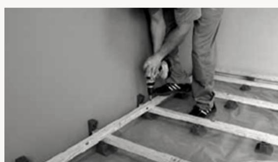
8. To ensure the planks are aligned in a straight line, install a stop strip approx. one plank width + 10–15 mm from the wall.
