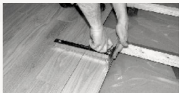
3. Use a tapping block during installation.
