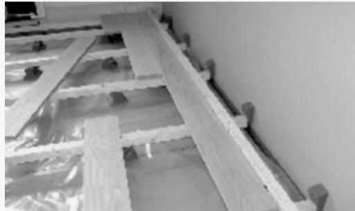
1. Start by laying the first plank against a straightedge. Planks should be nailed with a nail gun at a 45° angle. Glue all end joints. See point 11 for choice of fasteners.
