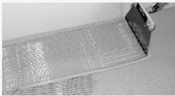
2. Apply HØRNING MS Flexlim with trowel no. 6. Approximately 1 litre per m<sup>2</sup> should be applied. Do not apply more adhesive than can be installed within 20 minutes. Installation must be carried out in wet adhesive. Adhesive must not be forced up between the planks, and tongue and groove must not be glued.
