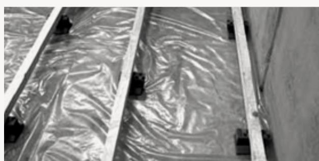
3. Lay the first row of joists with a 50 mm clearance from the wall. The joists should be put down with a centre distance depending on the floor load level.
