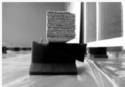
1. Putting joists on chocks can be done using plastic blocks and wedges. In case of risk of rising moisture from the subfloor, a 0.2 mm plastic sheet should be laid and taped with a 20 cm overlap.
