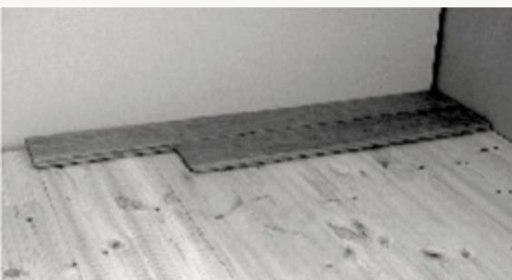
3. Remember to put down floor paper between the two floors (only when screwing) to avoid creaking. Planks should be installed in the opposite direction to the existing floor.
