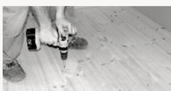
1. The subfloor must be stable and free from creaking. If necessary, re-screw.
