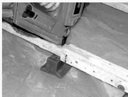
5. Secure the chocks to the joists with nails. Nail vertically or diagonally into the joist.
