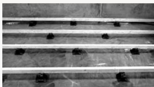
2. The chock distances for floor joists depend on load level, joist dimensions, and joist type (sawn/laminated joists). For private residences, offices, and light commercial use, the general chock distances apply to sawn softwood joists. At joist ends, chock distances must be reduced by 10%. **See point 7 and 12 above for distances.**
