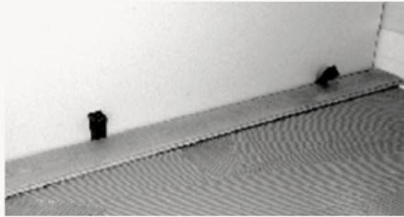
3. Use wedges to adjust the alignment of planks in the first row.
