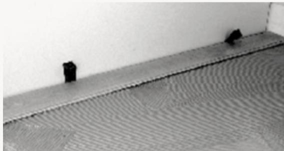
1. Use wedges to adjust the alignment of planks in the first row.
